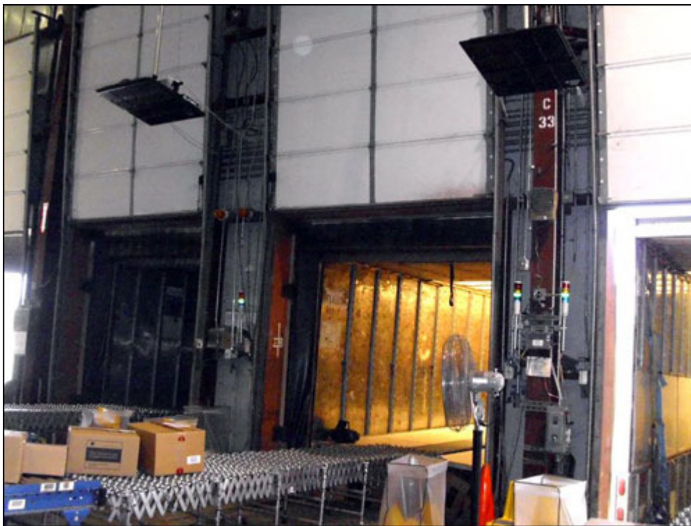
The system tracks the movements of pallets, boxes and bags through loading dock doors and into the backs of trucks.
